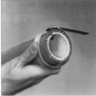
Tighten clamps in the same direction as the helical wire.
